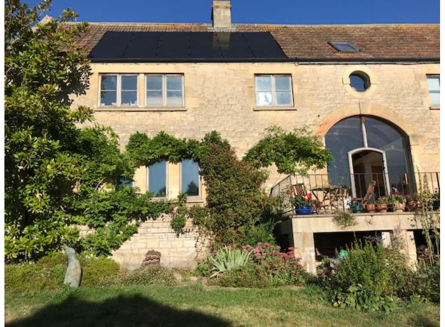
In-roof solar panels
