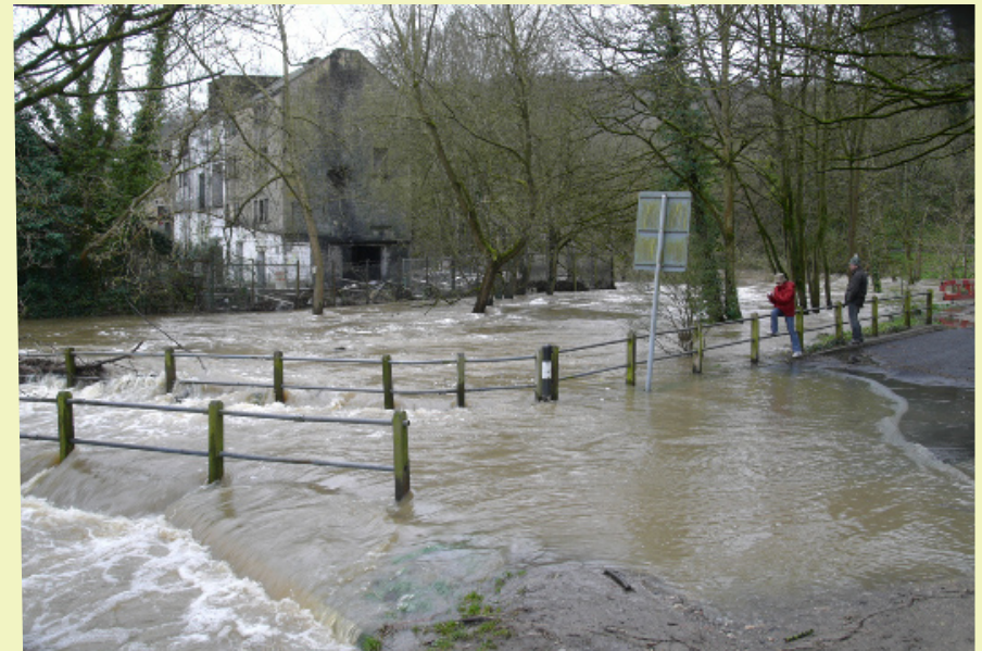
Freshford Mill and the flood plain in spate
