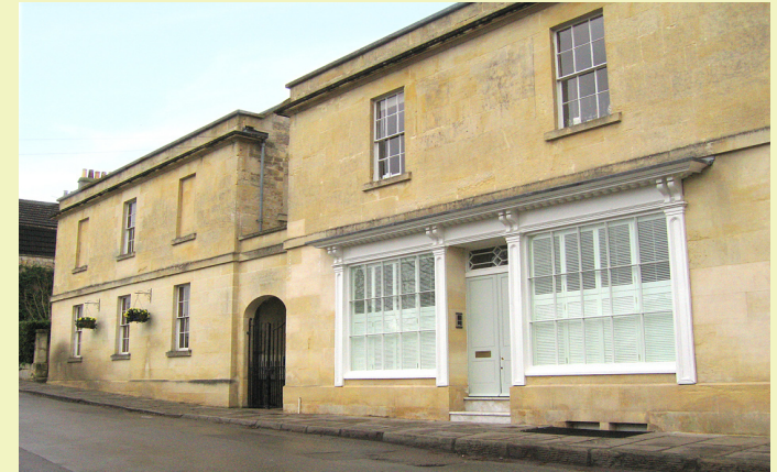
The Old Bakery (far building) with a former retail shop in the foreground
