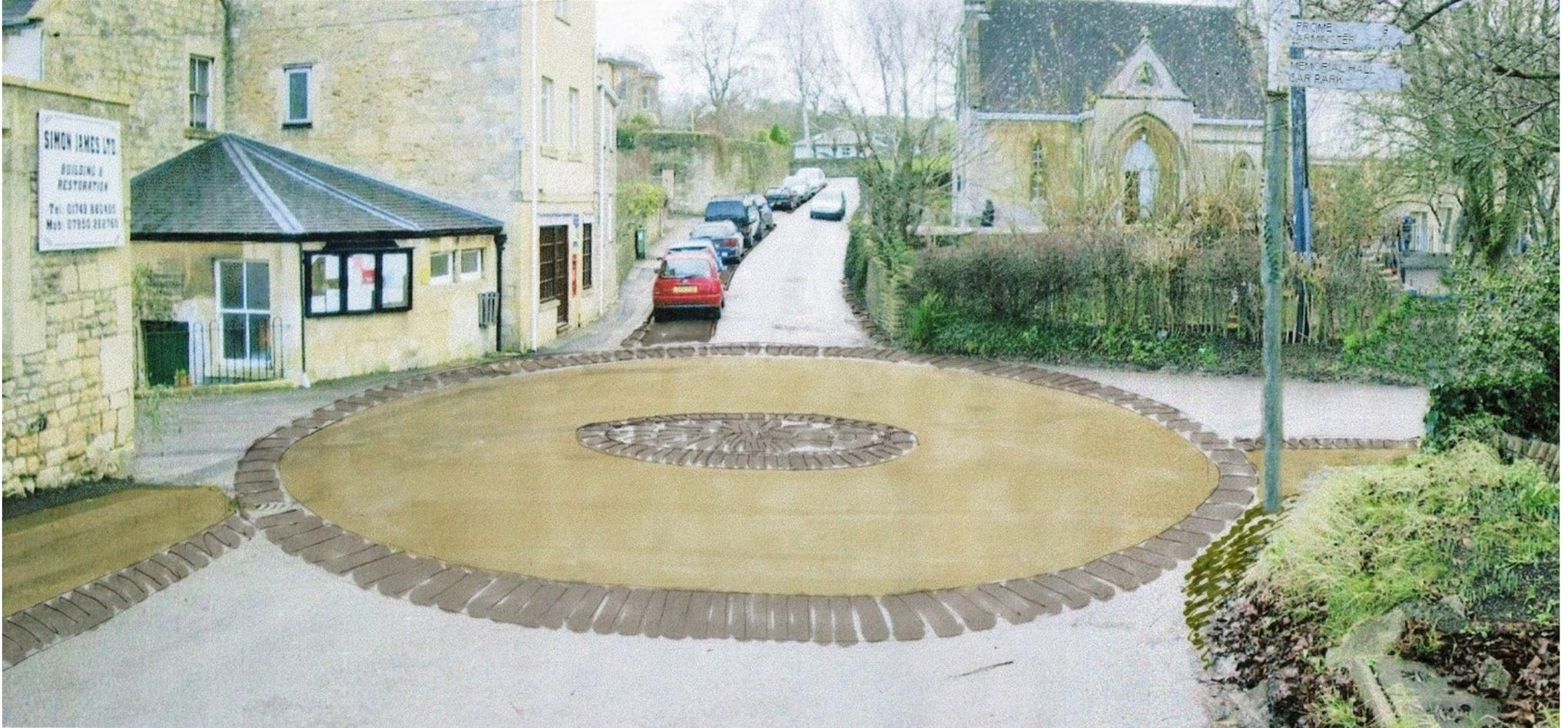
Other junctions throughout the village could be designed to emphasize the main road network and discourage unnecessary driving through the minor roads.
