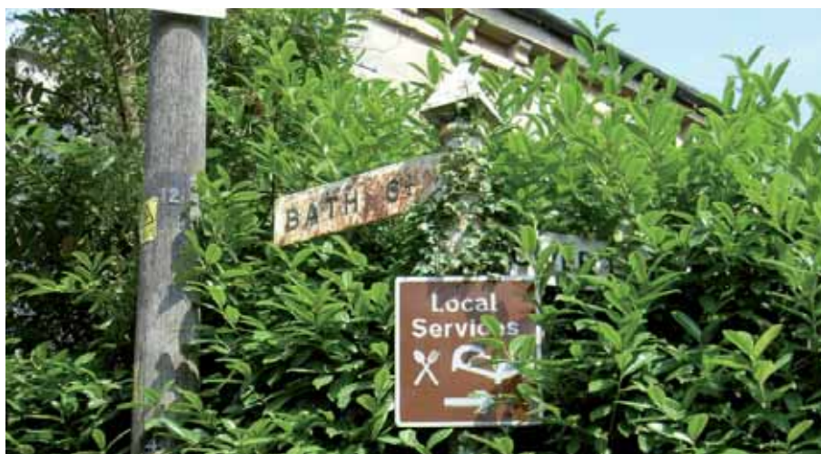
Cast iron finger-posts would benefit from restoration in some cases
