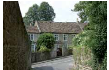
Traditional stone tiles contribute to the attractive roofscape in Freshford
