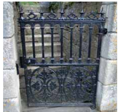
The diversity of building types and decorative details adds to the special interest in the area
