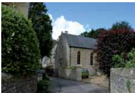
The use of local limestone gives Freshford a distinct sense of place
